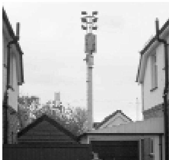
This Orange GSM and 3G, and Vodafone 3G and GSM are just two of eight base-stations at Worthing Football Club, a small ground surrounded by dense residential property. Floodlights are a favourite shared support for mobile antennae. BT helped sponsor the new lighting towers that now bear the antennae.
